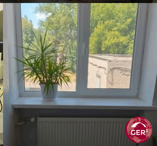
"GER3 replaced the heating system at the Diagnostic Centre of a hospital in Khersonska oblast, benefiting some 11,511 people. © Global Emergency Relief, Recovery and Reconstruction (GER3)
